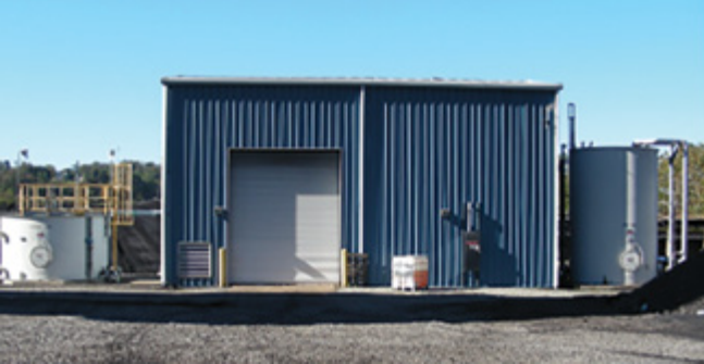
Figure 29. Clairton Plant's Coal Storage Area storm water collection and treatment system include solids and metals removal and pH adjustment prior to discharge to the Monongahela River.
