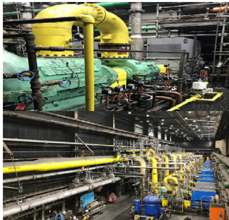
Figure 21. Axial Compressor Vibration Monitoring System.
