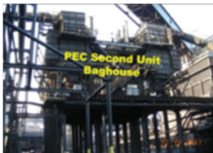
Figure 14. PEC Baghouse Infrastructure and PEC Baghouse Batteries 13–15 showing the coke guide enclosure, PEC hood and 13–15 & 19–20 PEC, or second unit, baghouse.
