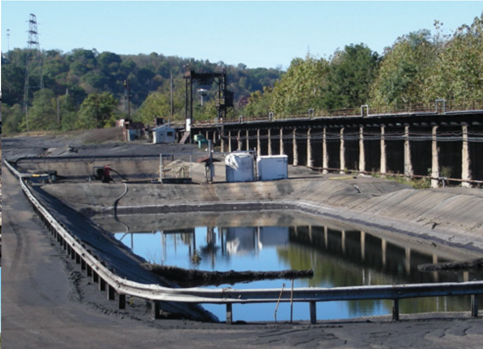
Figure 29. Clairton Plant's Coal Storage Area storm water collection and treatment system include solids and metals removal and pH adjustment prior to discharge to the Monongahela River.
