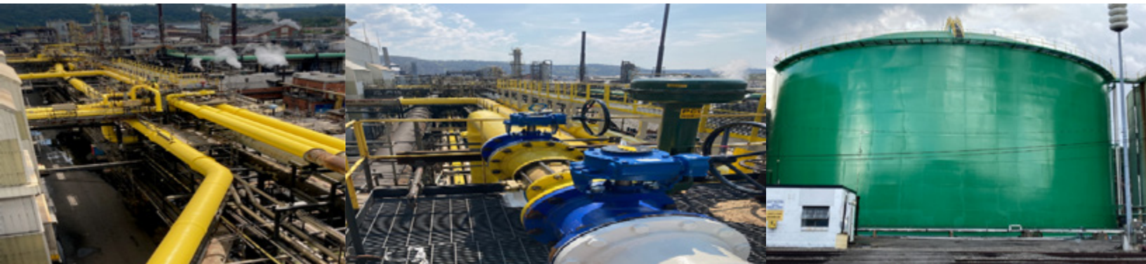
Figure 19. By-Products Piping and Tank Improvements.
