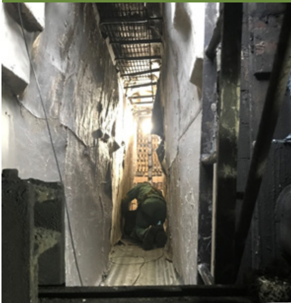
Figure 12. Regenerator Cleanout in Progress.
